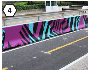
Concrete "Jersey" barriers
